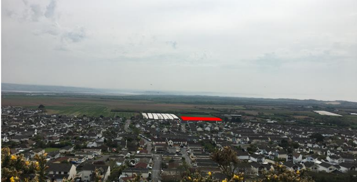
Photograph of Great Field setting from Fairlynch Lane (site marked red)
