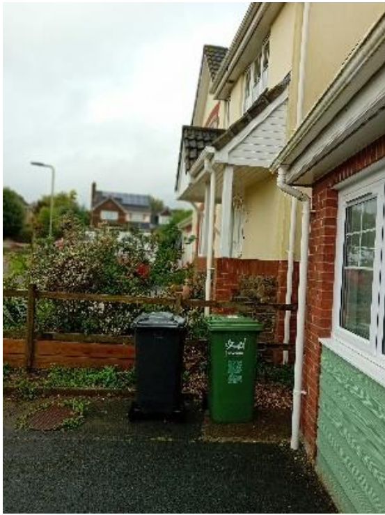
Figure 3. Existing porch viewed from the south.
