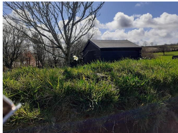
Existing Shed on Site
