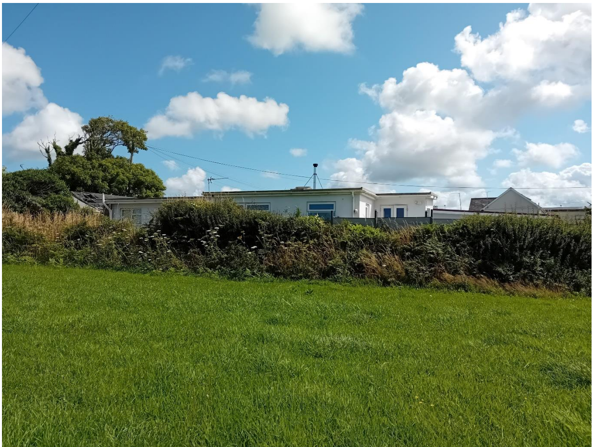
Field level view of No. 5 and 6 Fortescue Bungalows
