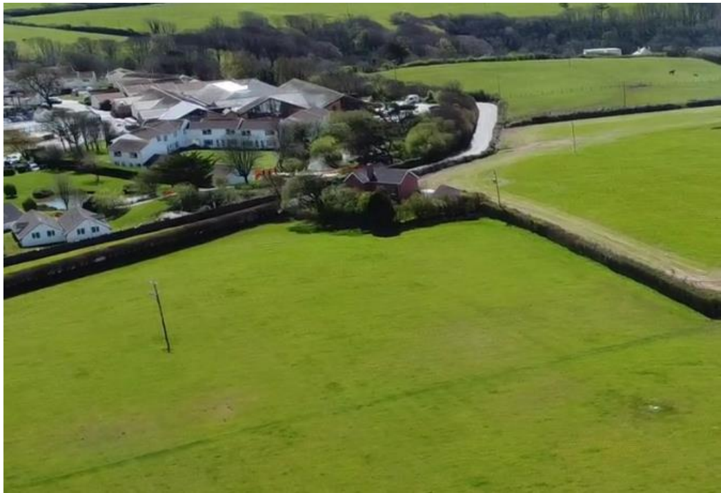
Drone View of Landscape House
