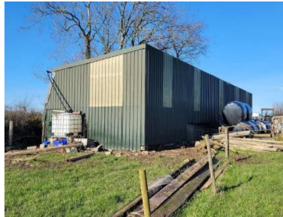
Existing site photo
