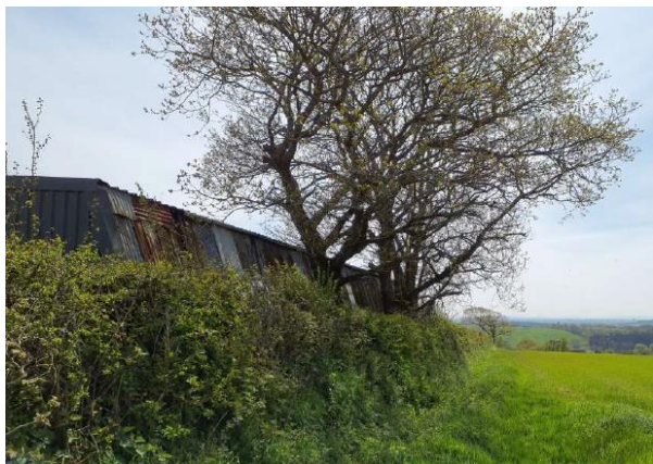
Existing site photo
