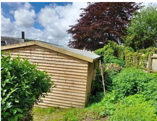
Rear of dining shelter and boundary with number 18 The Orchards
