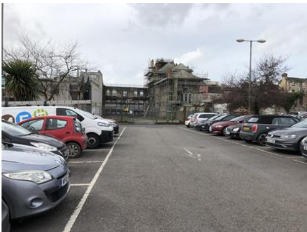
Rear of application site viewed from Queen Street car park
