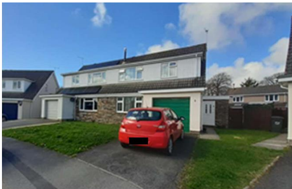
Front elevation of dwelling
