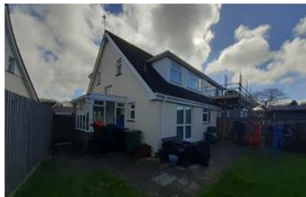
Rear elevation of dwelling
