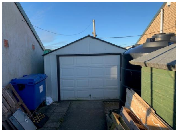
Existing buildings to be replaced
