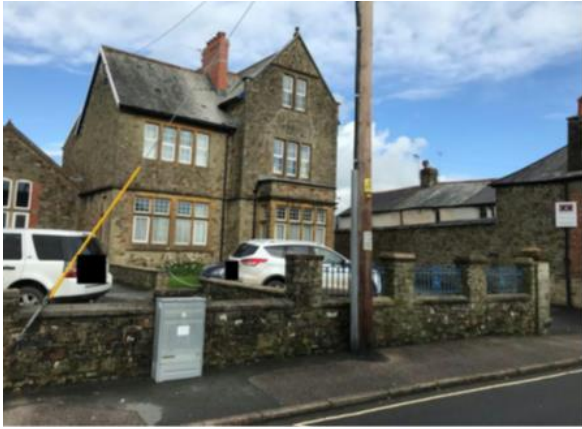
Front of building
