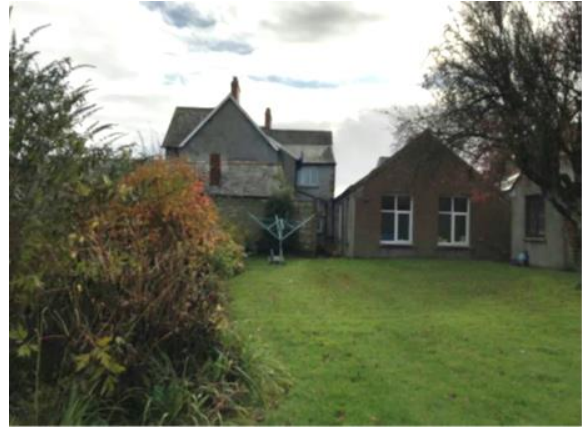
Rear of building garden and garages
