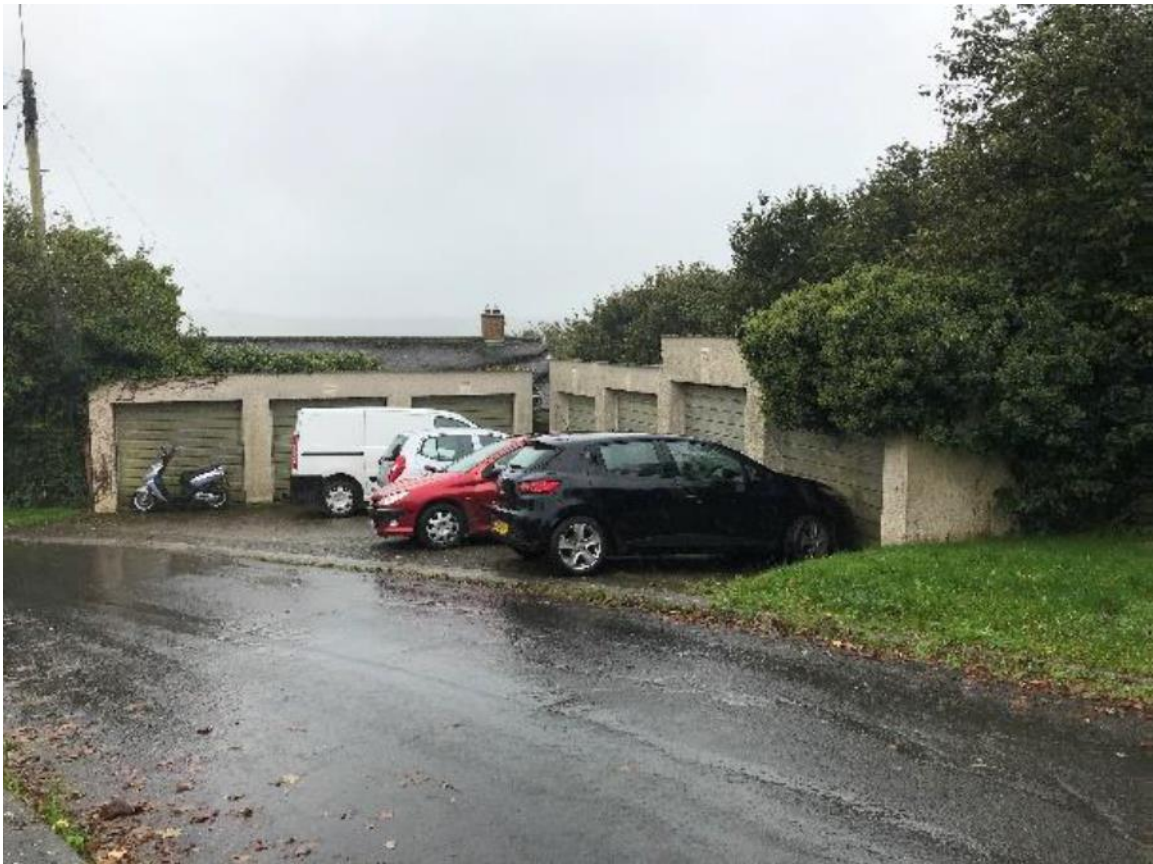
Existing garages to south to be demolished (Plot 2)
