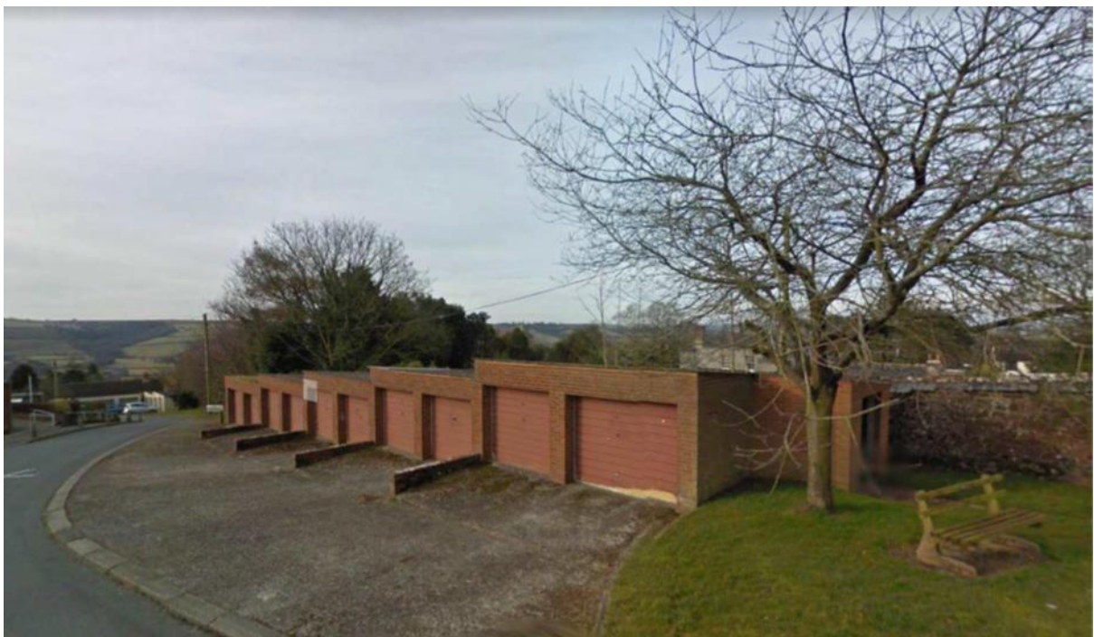
Existing block of garages to be demolished (Plot 1)
