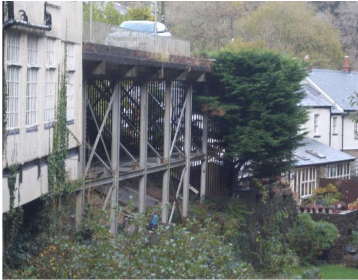
Photograph 1 shows a view of the elevated car park from footbridge
